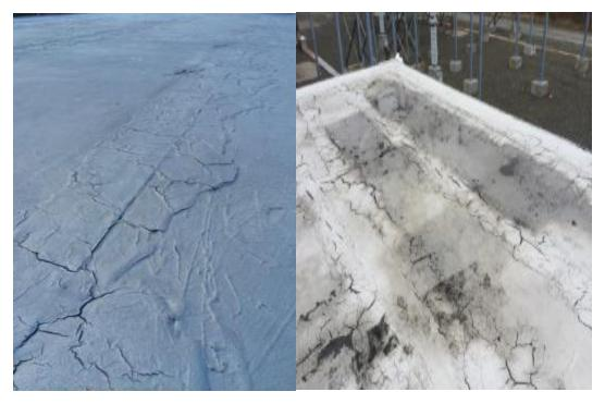
Figure 15: Terminal Station Control Buildings (Come By Chance and Sunnyside) showing cracking and deterioration of the roof membrane systems.
