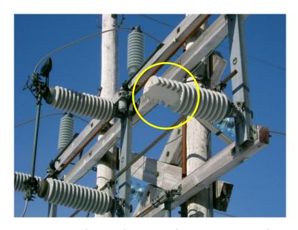
Figure 4: Broken Insulator on 69 kV Disconnect Switch
