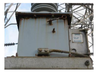
**Figure 2: Rusting on Potential Transformer**
