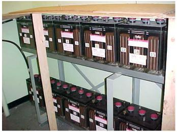
Figure 11: 125 V Direct Current Terminal Station Battery Bank
