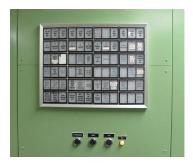
Figure 18: An annunciator commonly found in Hydro's terminal stations
