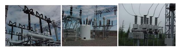
Figure 9: Circuit Breakers – ABCB (left), Oil (middle), and SF<sub>6</sub> (right)
