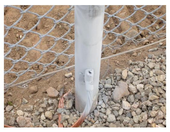
**Figure 7: Typical Grounding Connection on Terminal Station Fence**
