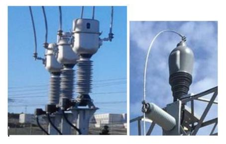
Figure 1: 69 kV Current Transformer (left) and Potential Transformer (Right)
