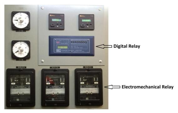
Figure 17: Digital and Electromechanical Relays
