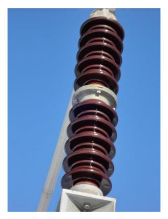
Figure 6: A Multi-cone type insulator prone to failure due to cement growth
