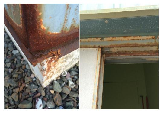
Figure 16: Building exterior cladding and doorways displaying severe rusting and deterioration
