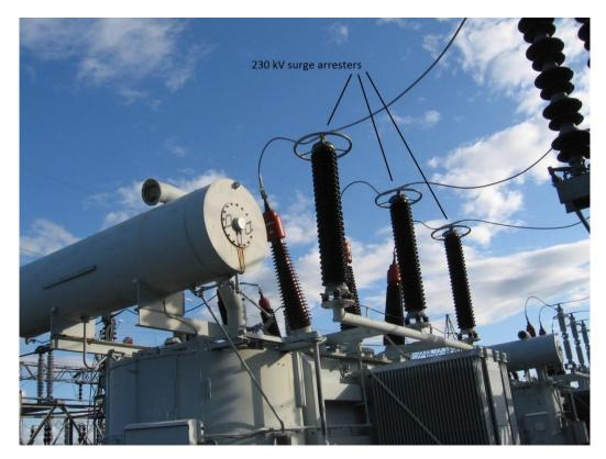
Figure 5: Western Avalon Terminal Station Transformer T3 230 kV Surge Arresters
