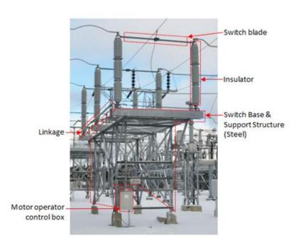
Figure 3: Various Components of a High Voltage Disconnect Switch
