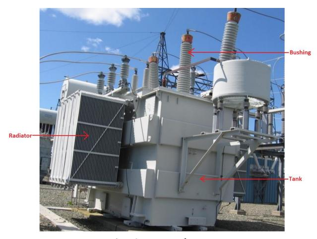
Figure 8: Power Transformer
